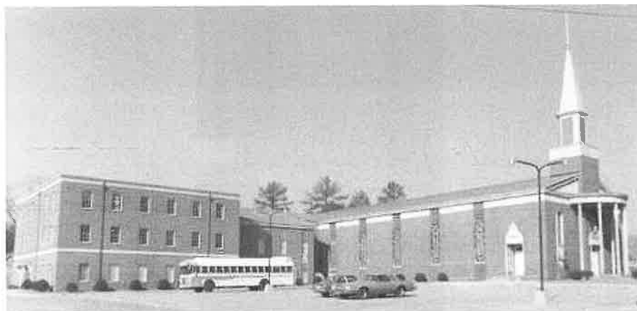
The south wing of Pleasant Ridge, completed in 1970
